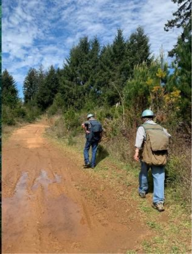
South of Mill Creek, flat road segments are difficult to drain.
