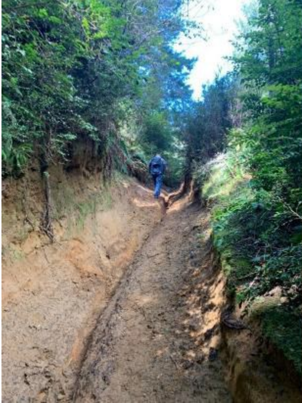
Unusable road segment North of Mill Creek Crossing Road Point 1.7
