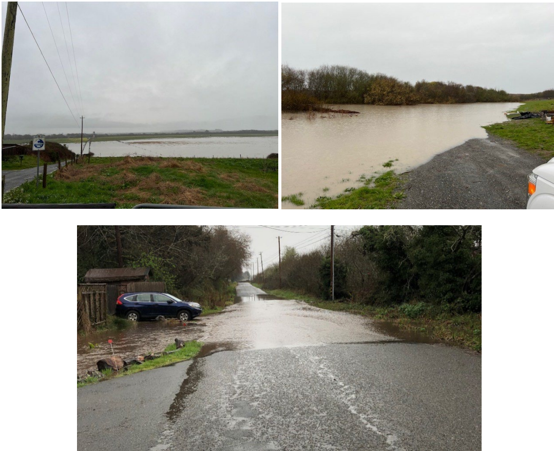
Figure 26: McKinleyville Flooding Impacts
